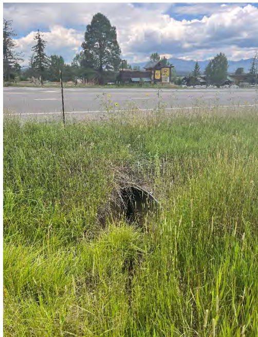
Photo 20: Culvert that drains wetland area D.
