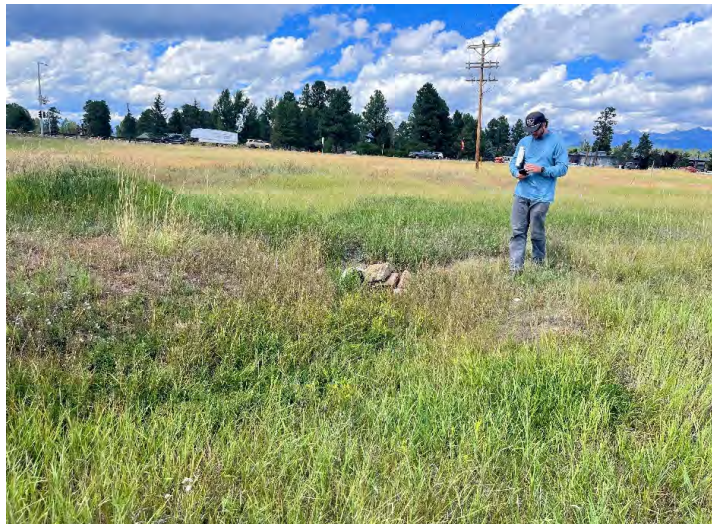
Photo 10: View of culvert northeast of Area B.
