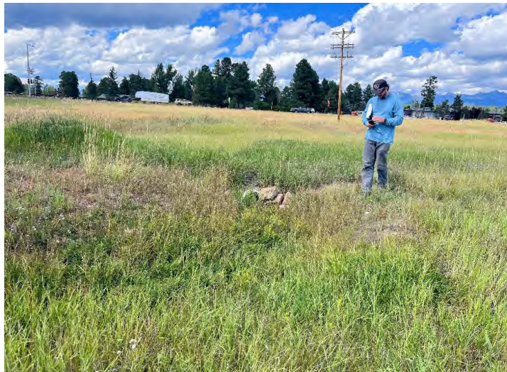
Photo 10: View of culvert northeast of Area B.
