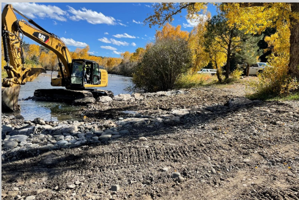
Boat ramp construction on San Juan near Pagosa Springs
