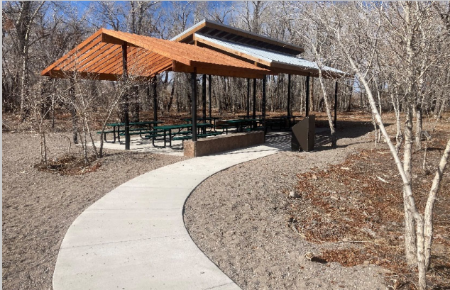
Freshly constructed shade structure and riverwalk trail for Riverfront Park in Del Norte on Rio Grande River
