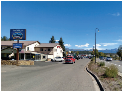
Figure 4.2 Current Condition of North Frontage Road
