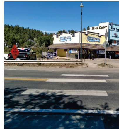
Figure 4.3 Existing Western Crosswalk
