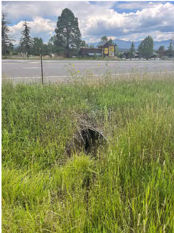
Photo 20: Culvert that drains wetland area D.
