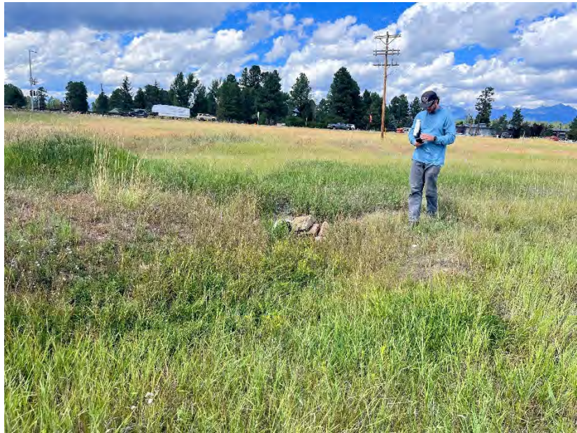
Photo 10: View of culvert northeast of Area B.
