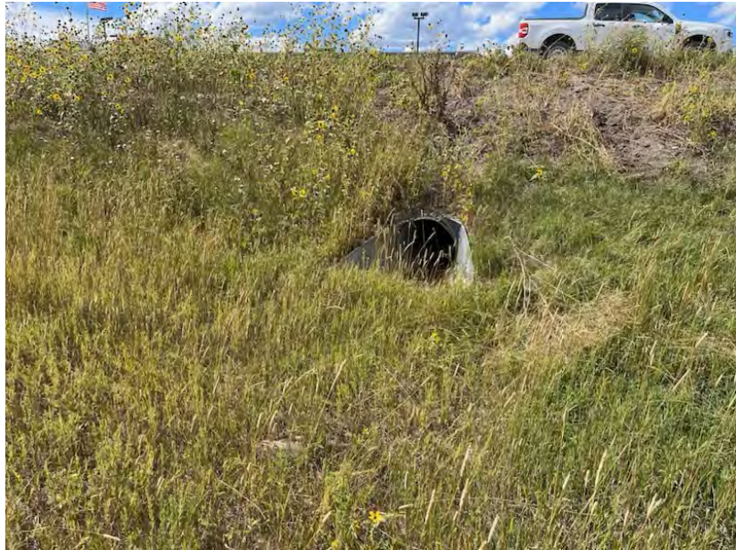
Photo 15: View of culvert on north end of Area C.
