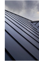
STANDING SEAM METAL ROOF
